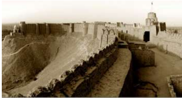
Figure 4. The defensive wall of Kot Diji Fort Sindh, Pakistan.
