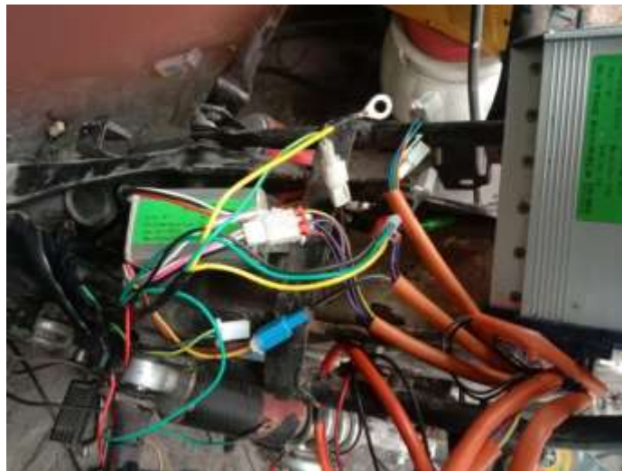
Fig.8 Wires connection with Motor
