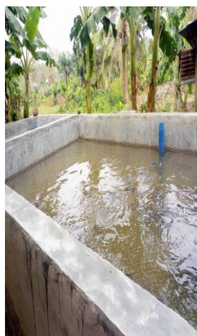
Figure 1b Concrete fish pond
