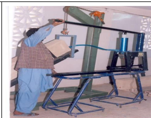
Figure 5. Forced grouting of cement Slurry for baked clay beams.
