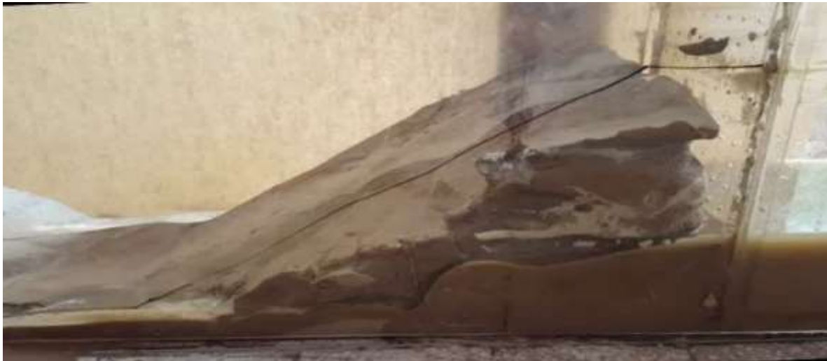
Figure 4. 2: Slope after failure
