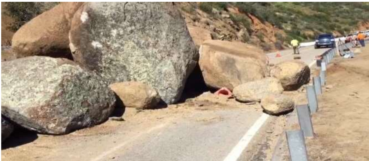
Figure2. 3: Example of rock fall
