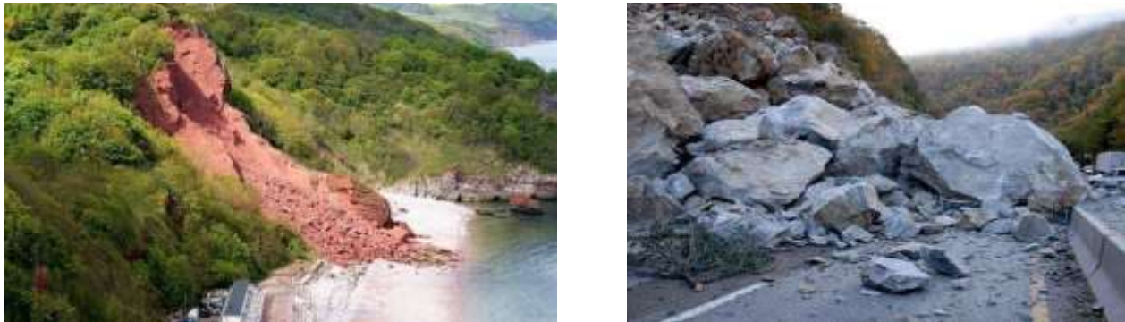
Figure2. 2: Example of Landslide and Rockslide
