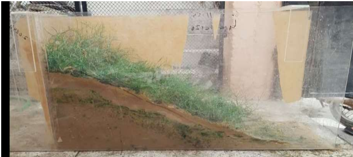
Figure 4. 3: Slope before failure with vegetation cover
